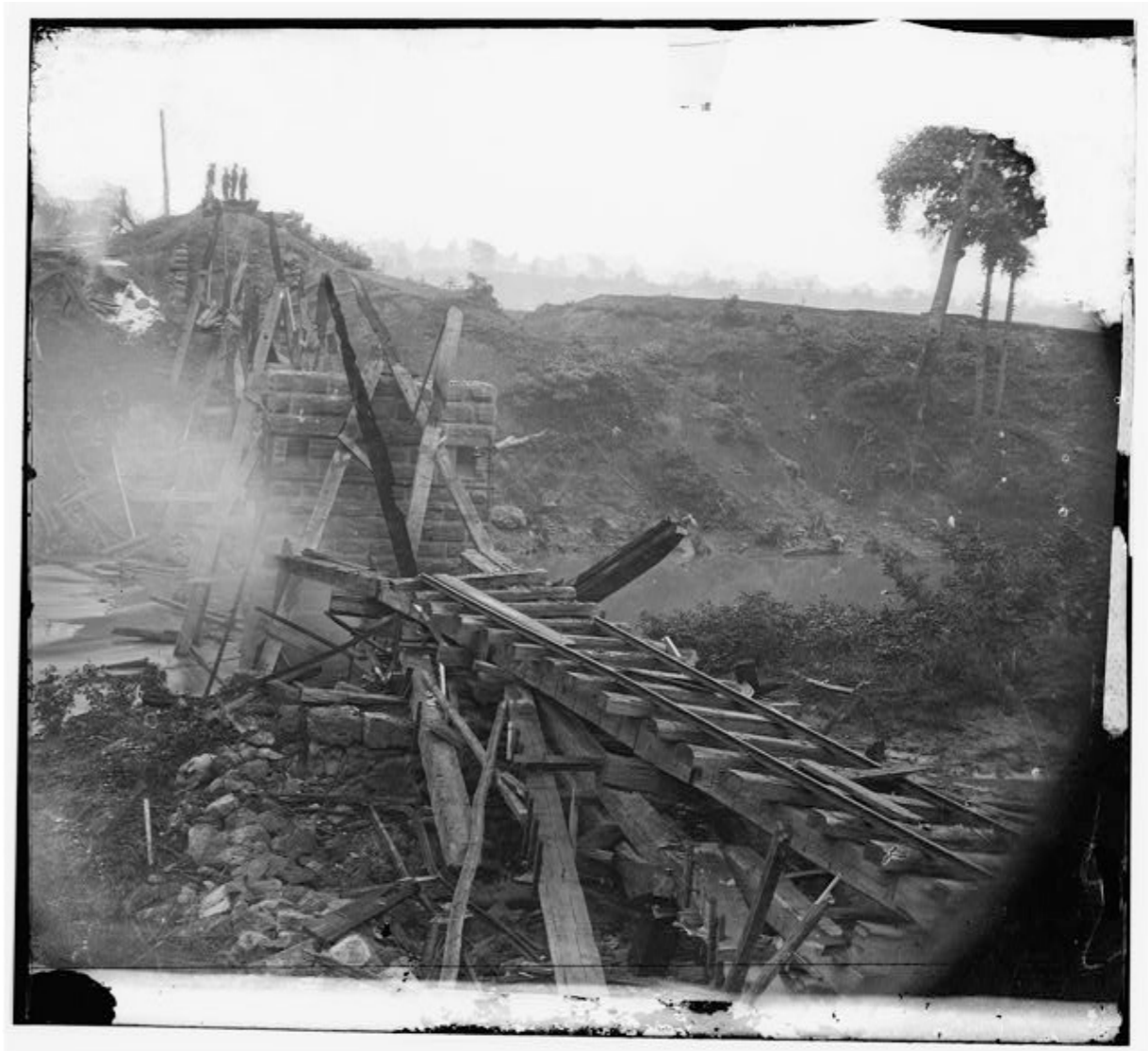
A destroyed railroad bridge over the North Anna River on the Richmond and Fredericksburg Railroad.
